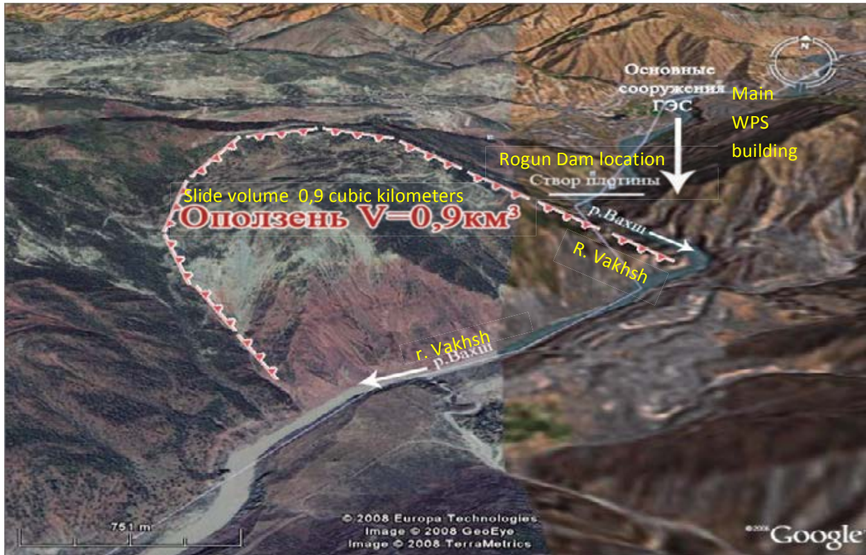
Figure 10. Tremendous slide of volume 0.9 cubic kilometers over the tail water basin of the Rogun dam 148
