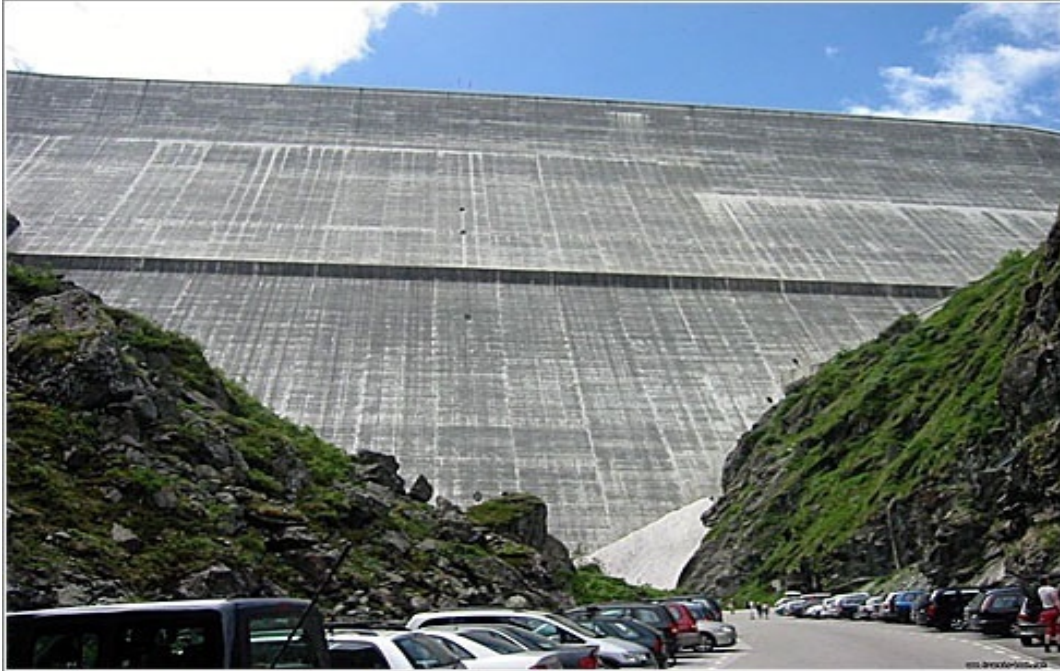
Figure 11. Incomplete wall of the Rogun dam – at 35% of the designed height 149
